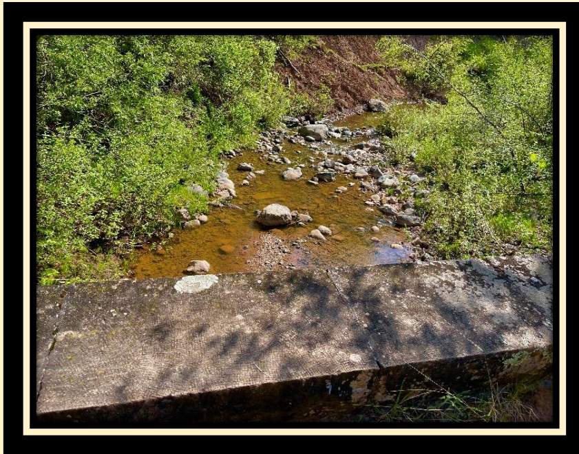
View from bridge three, photo spot #2
