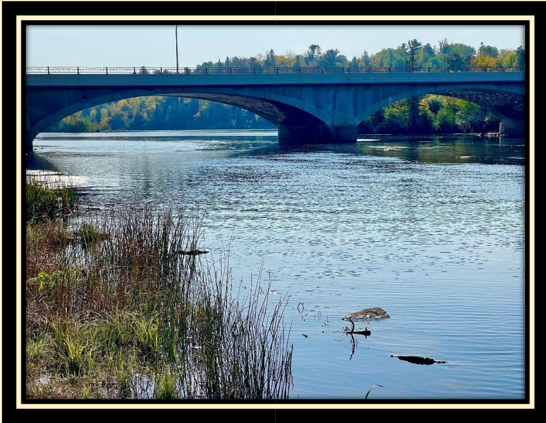
View of the historic Biauswah bridge, photo spot #1
